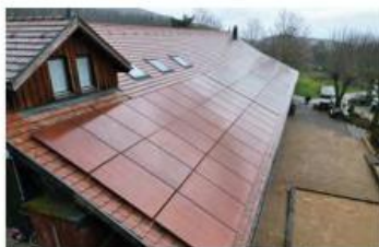
Panneaux bruns, implantation en rive Jungholtz (68)
